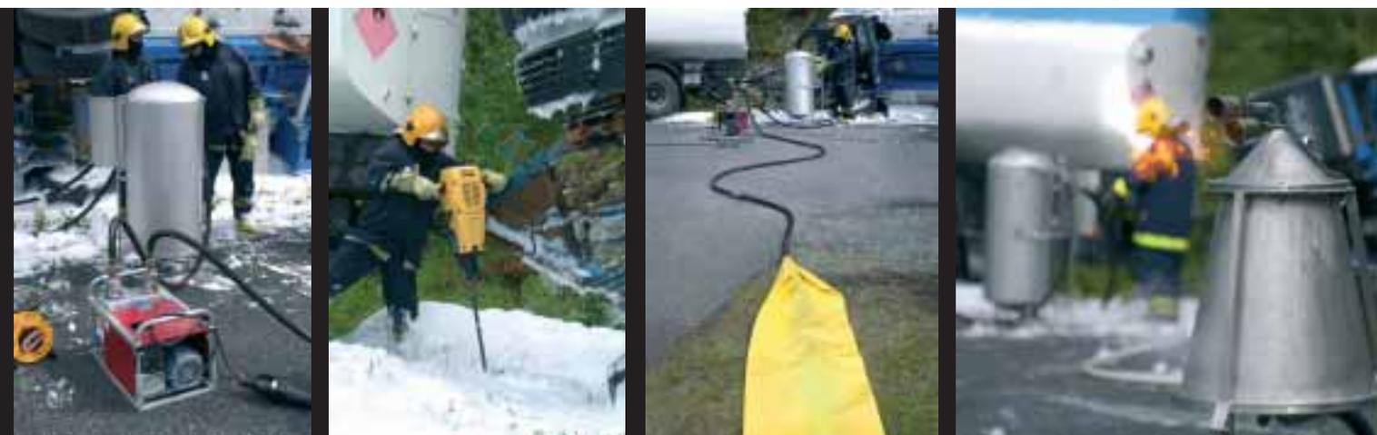
The process is based on powerful vacuum suction, by means of which volatile hydrocarbons - such as petrol - can be recovered from the ground as both liquid and vapour by means of suction tubes inserted into the ground.
